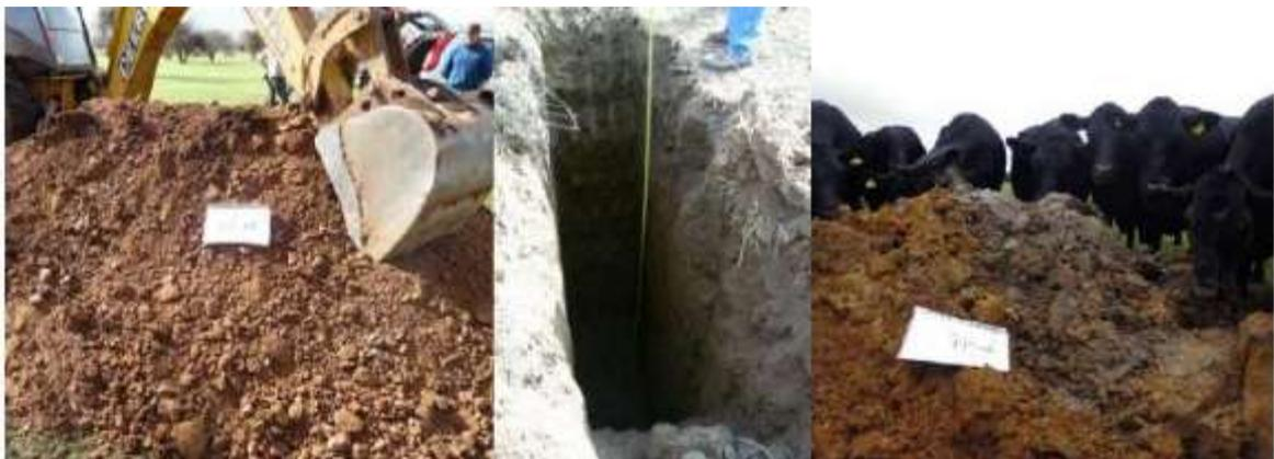
Fig. 3: Trial pit detail for geological log and sampling
